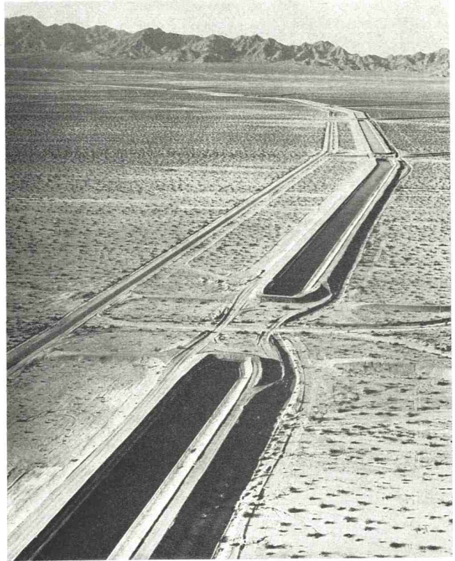
DESERT WATERWAY—Section of Colorado River Aqueduct canal on its way to Southern California coastal plain. The canal is 55 feet wide at the top, slopes to a bottom width of 20 feet and is about 10 feet deep at the center.
