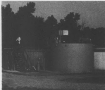
Wastewater testing facility, Chelsea, Michigan.
